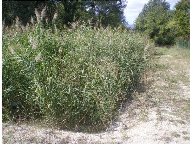
**Figure 4:** Filtration basin for the treatment of water from a small town in France<sup>6</sup>
