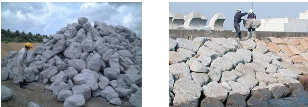
**Figure 5:** Frontier rock™ (left) and restoration of quay (right) with Frontier rock™
