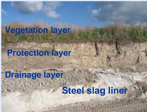
Landfill top cover with steel slag liner
